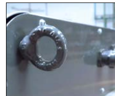
Detalle anclajes. View of fixtures.
